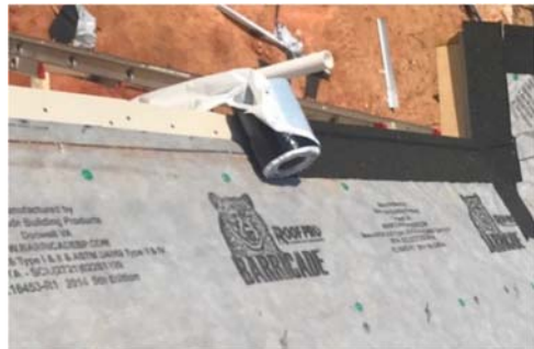
Sample Photo 6: Drip Edge with Self-Adhering Starter Strip
