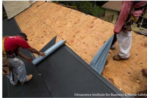
Sample Photo 4: Underlayment "peel-and-stick"
