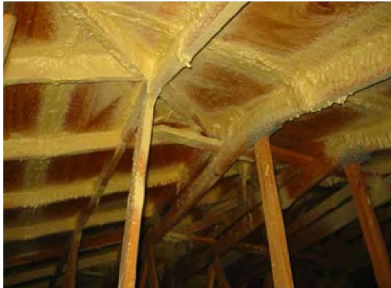
Figure 1. Closed-cell spray polyurethane foam adhesive applied to the underside of the roof sheathing at the joints between the sheathing panels and along all intersections between roof sheathing and all roof framing members.
