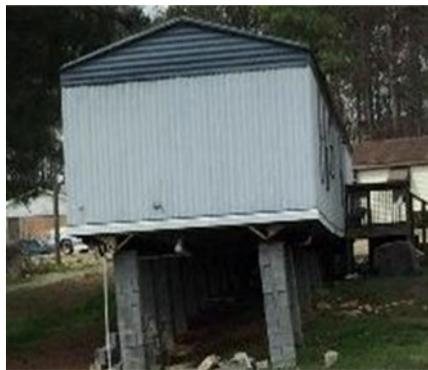
*Figure 3. Ineligible dry-stack foundation.*
