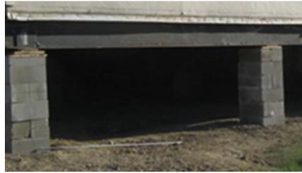
*Figure 1. Ineligible dry-stack foundation. No mortar is seen between the blocks.*
