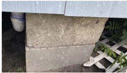
*Figure 2. Ineligible dry-stack foundation.*
