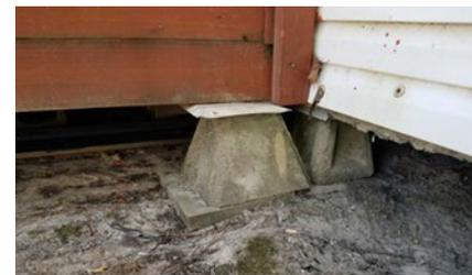
*Figure 4. Ineligible dry-stack foundation.*
