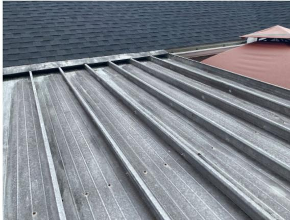
Figure 4. Example of accessory roof that meets main roof at eave.
