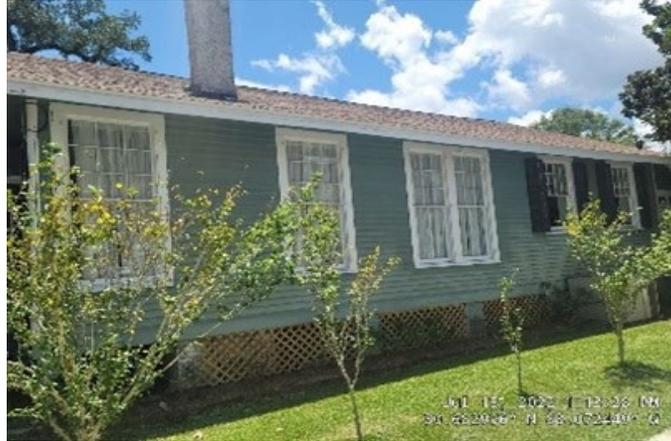
Figure 3: Example of skirting on home built to the HUD Code
