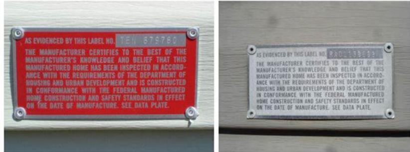
Figure 5: Examples of HUD Label on home built to the HUD Code
