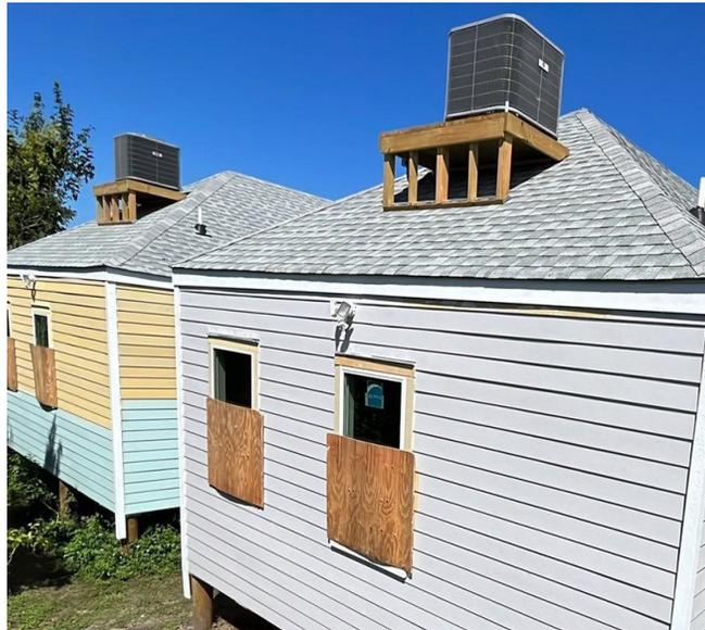
Figure 1: Wood framed supporting platform built over the roof area of a home
