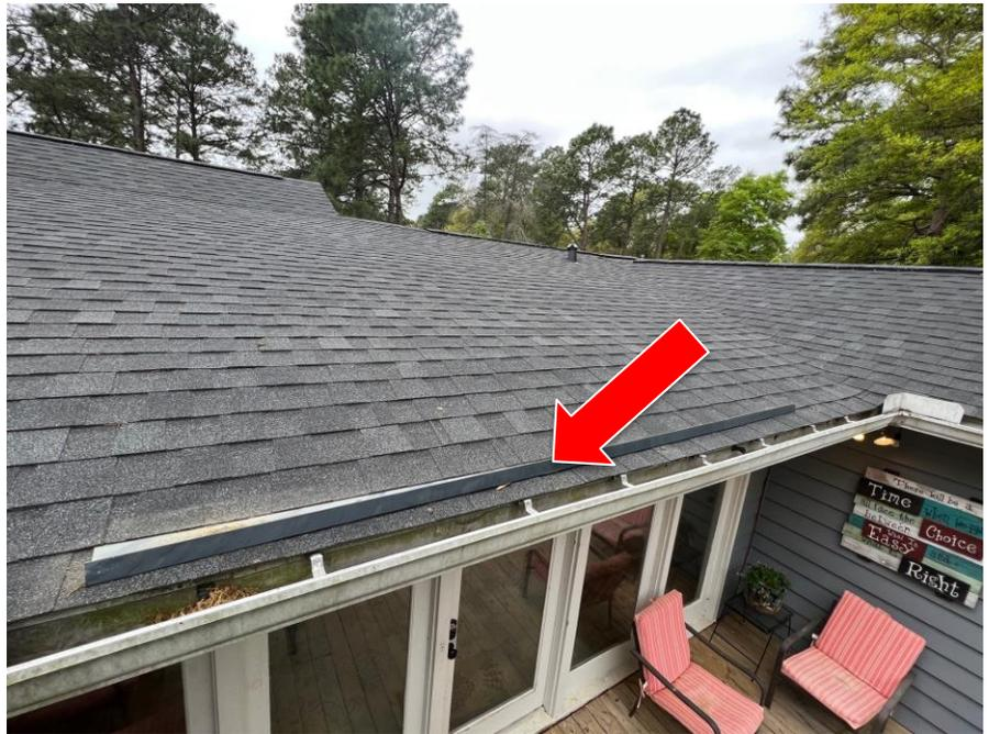
Figure 1: Example of rain diverter installed on asphalt shingle roof.
