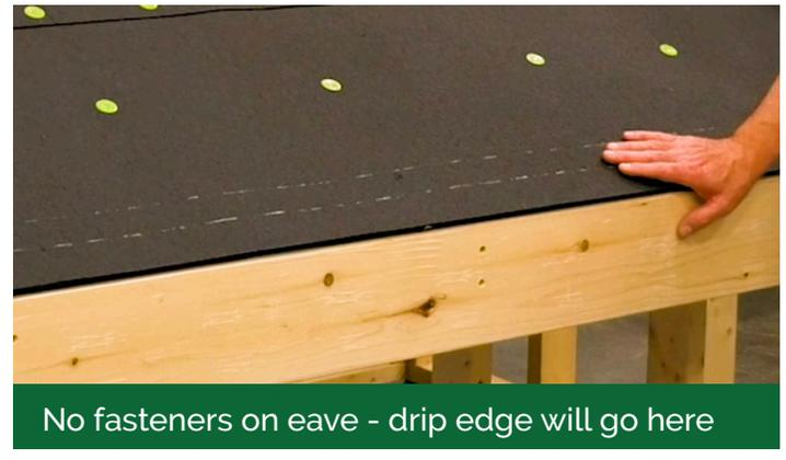
No fasteners on eave - drip edge will go here
