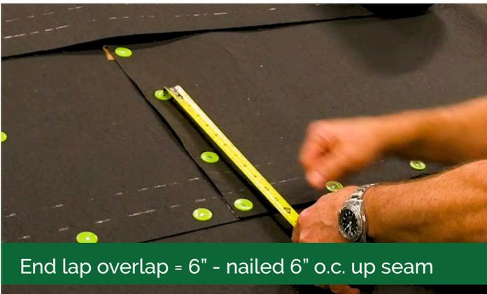
End lap overlap = 6" - nailed 6" o.c. up seam
